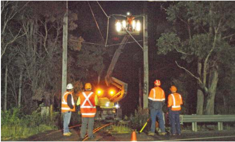
The mobile tower platform is used to make the final adjustments around 3:00am.
