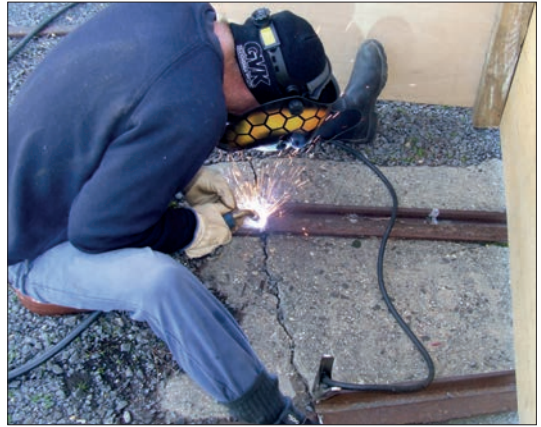
Frank Schroeders welding one of the broken rail joints on the Carbarn fan. Jacqui Smith
