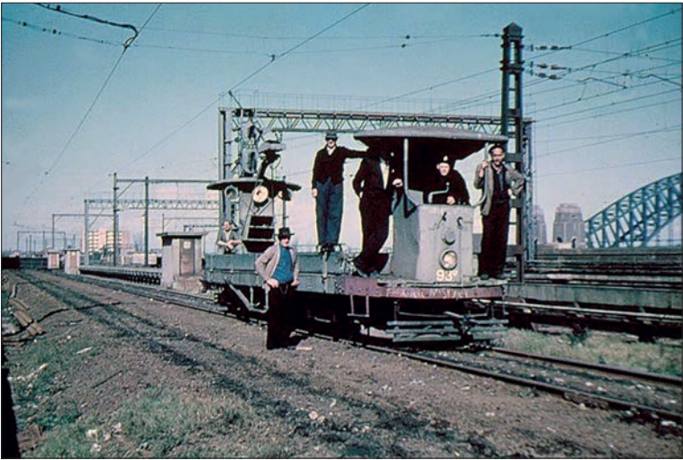
The last trams to run on the bridge were four U class ballast cars which were used in track dismantling after closure. With the southbound track already lifted, 93u poses near North Sydney Station in July 1958. Sydney Tramway Museum
