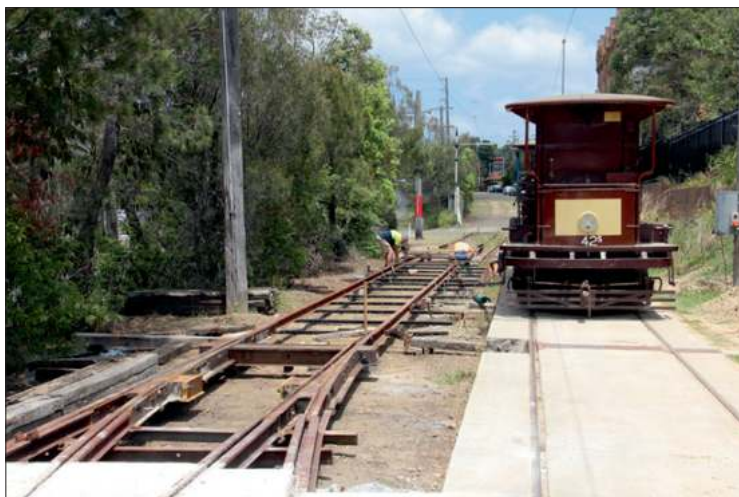
Progress on the relaying of the eastern track north of Pitt Street on 4 November. The new cross box and cover are in place and steel angle iron sleepers are being installed in preparation for concreting. Martin Pinches
