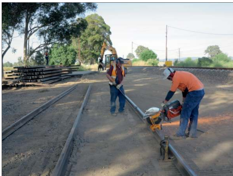
Richard Gilbert holds the rail steady whilst Alastair Reither cuts another 13-metre length on 22 November. This was done for almost four kilometres of rail.
