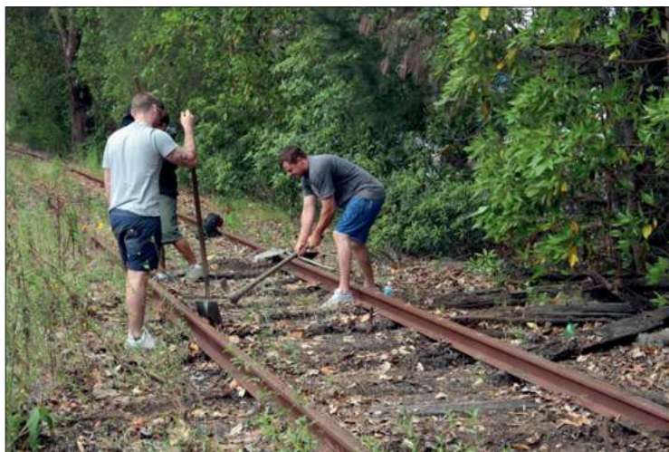
CSO workers removing rotted sleepers from the track up Army Hill from the army depot level crossing to the northern terminus on 10 November. Martin Pinches
