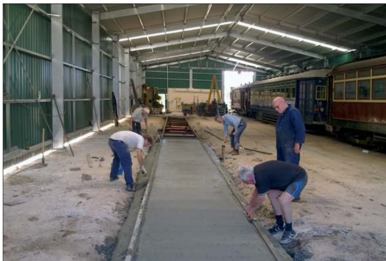
Road 4 in the new shed and the walkway to the left being prepared for concreting on 1 December 2012.
