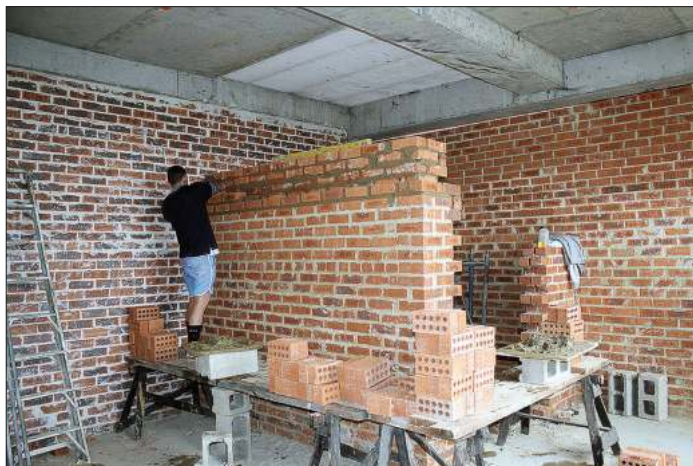
Bricking up around the future lift well in the YMCA building on 21 July. Martin Pinches
