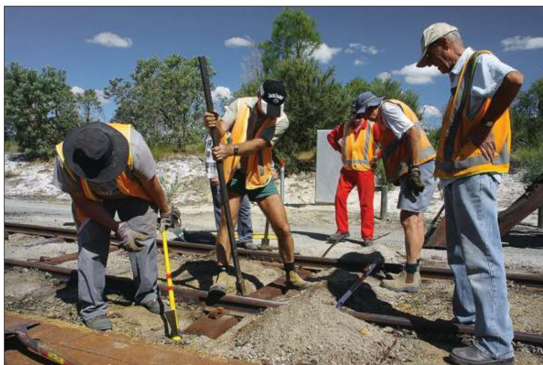
The track team at work near the Village road crossing on 14 April: Trevor Dennhardt fastens the rail clips on a steel sleeper as Nick Tsiaglis (left) and John Azzaro (in red overalls) hold the sleeper in place, Lindsay Richardson checks the gauge bar, and John Budd (right) is ready to start shovel-packing the sleeper.
