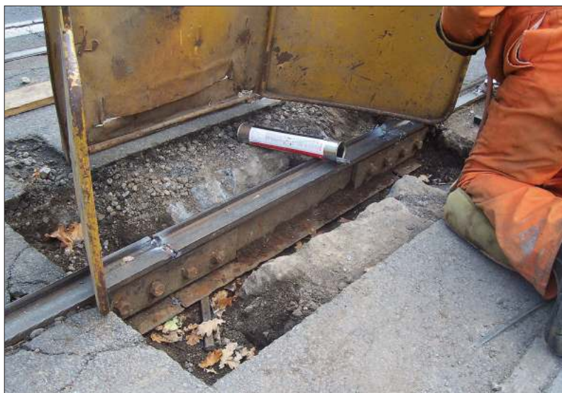
Another track joint receives attention. Our workers have almost lost count of how many sections of rail have been inserted to repair broken joints.
