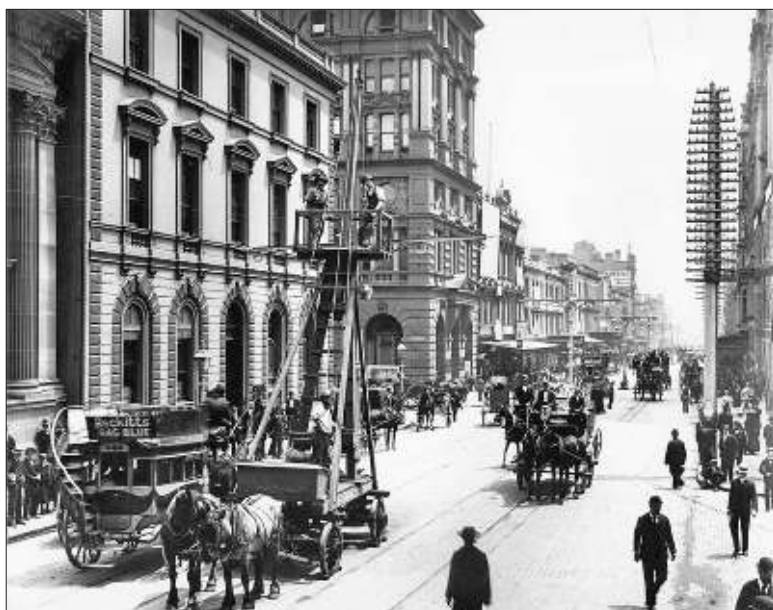
Erecting overhead poles in George Street at Wynyard Street.
