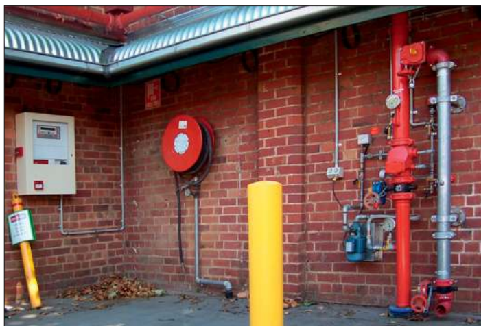
Modern sprinkler controls at the entrance to Bendigo Tram Depot. Operation of the sprinkler system is on the right, with the fire panel to alert the fire brigade on the wall on the left.
