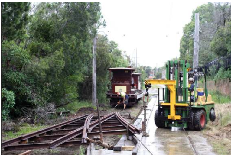
Ballast motor 42s assisted with moving the heavy pointwork into position using minimum manpower. This view is looking south to Pitt Street.
