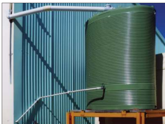
The new rainwater tank at the west end of the Oketon Geddes Carbarn, organised by Jack Kendall, with the supply connection to the Members' Room kitchen shown.
