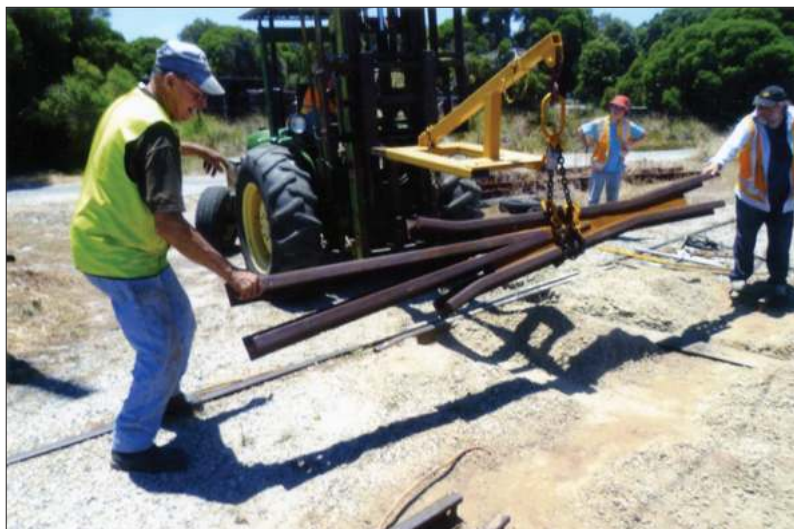
Jack Kendall and Kim Freind steady the repaired crossing for re-installation at the main line turnout to the Lindsay Richardson Car barn on 11 January
