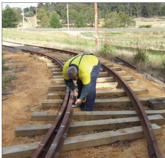
Kym Smith bolting the check rail to the inner rail on the south western curve. Jacqui Smith
