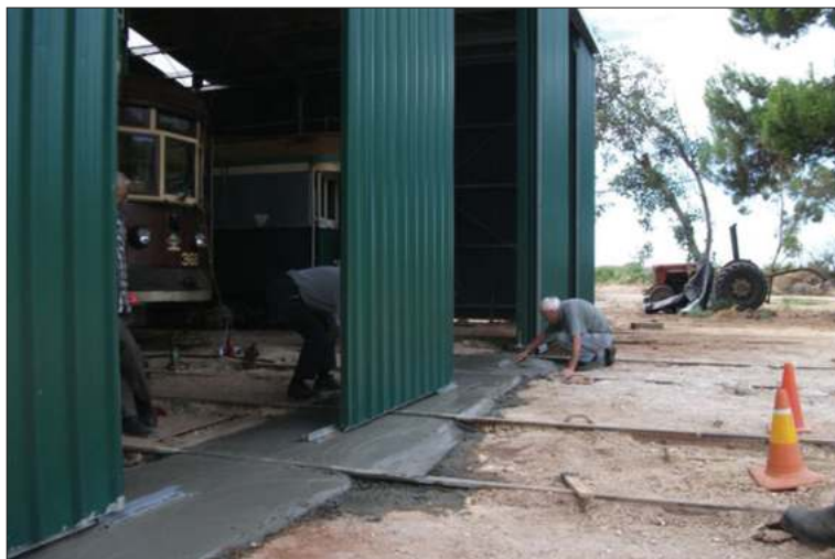
Laying the concrete at the doorways of the new shed in January 2012. Chris Summers
