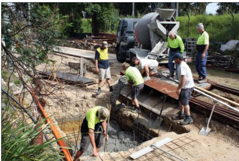
Concreting the pit to house the Sydney style under-track point changing mechanism on 14 April.
