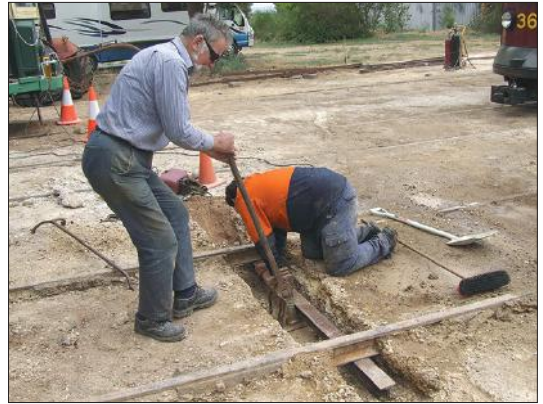
John Pennack and William Adams prepare an upturned rail 'sleeper' for welding under the raised track on Road 4. Kym Smith
