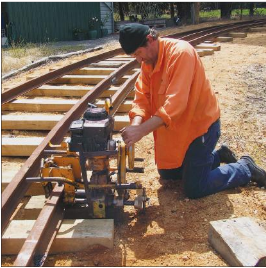
Anthony Smith drilling the bolt holes into the inner rail of the south west curve.
