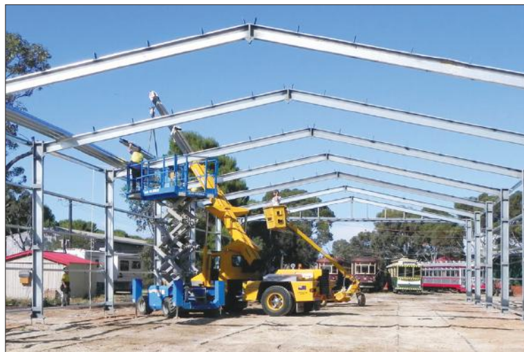
Contractors erect the shed frame on 9 November 2011, with trams in outside storage on the depot fan. Kevin Collins
