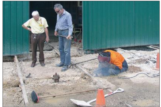
Mike Crabb explains the technicalities of welding to John Pennack while William Adams carries on with the task of welding the next rail 'sleeper' in place.
