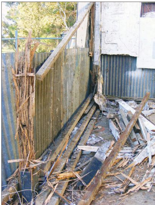
An example of some of the hidden white ant damage that was found once demolition began; the damage being far worse than was initially believed.
