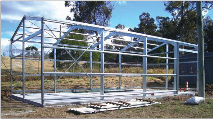
Construction of the new substation with the frame complete. Peter Hyde
