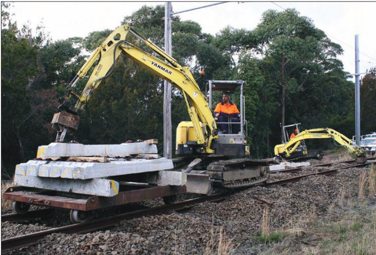
Concrete sleeper insertion commenced from the National Park end of the line on 31 August. One machine lifts the sleeper and places it beside the line. A second machine inserts the sleeper under the rails.
