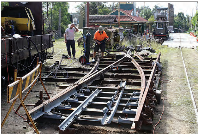
Construction of the new left-hand pointwork is progressing well.
