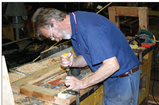
Rod Burland works on construction of new floor hatches for C 37 on 4 June.
