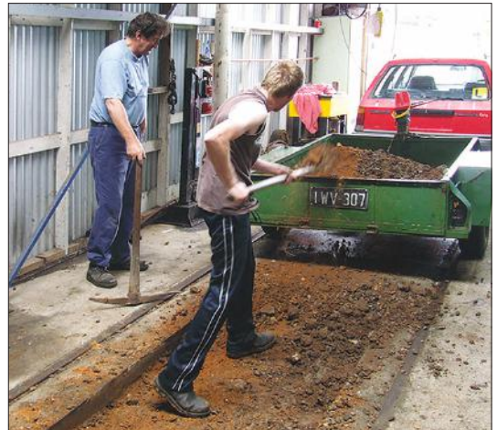
Anthony Smith and Daniel Edwards remove the dirt infill from between the rails in the Truck Shop.
