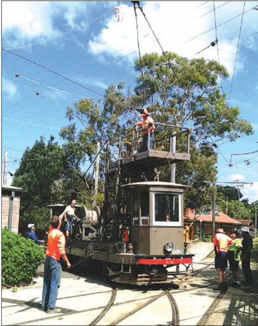
Erecting the Cross Street overhead wiring on 10 February. The wiring still requires tensioning work but it enabled trams to use Cross Street during the Tramway Festival. Ian Saxon
