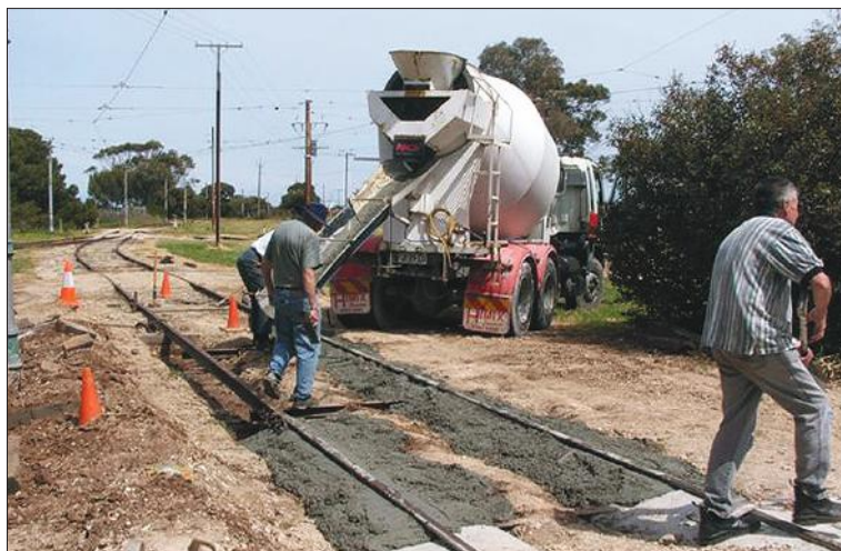
John Pennack, Michael Crabb and Charlie Rodgers spread the concrete for the first section of track at the yard throat on 30 September 2010.
