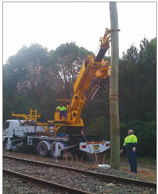
A new pole being erected on 11 August to replace pole 131 damaged during violent winds in earlier in the month.
