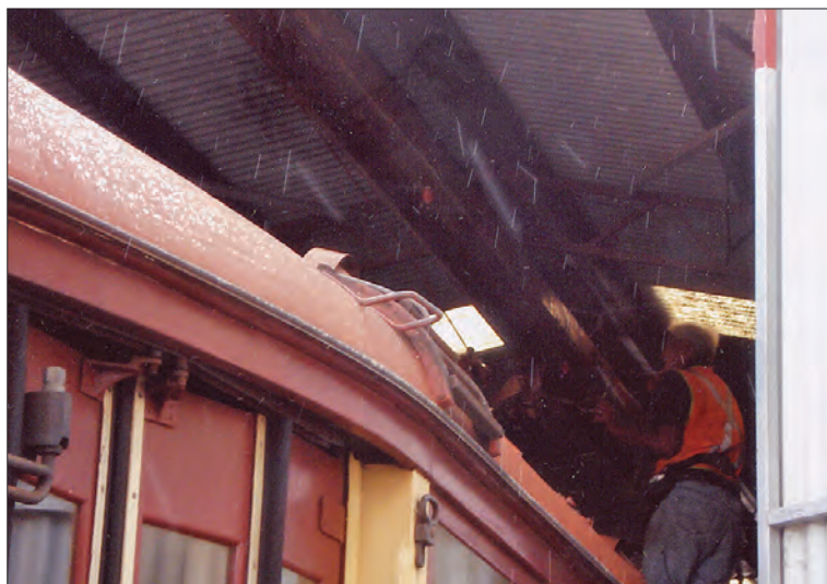
Duncan McVicar fitting the ears into the newly-installed overhead trolleying over the pit road track and Adelaide H 371 on 14 April.
