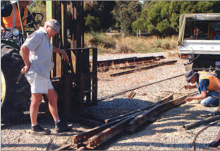
Noel Blackmore, watched by Graham Bedells, prepares for the lifting of the damaged crossing of the main line turnout to the Lindsay Richardson Carbarn on 7 April. John Azzaro is operating the forklift. Lindsay Richardson
