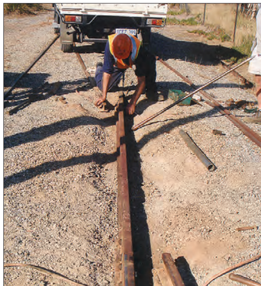
John Azzaro (left) and Graham Bedells fitting the temporary straight rail in place of the removed crossing on the main line turnout to the Lindsay Richardson Carbarn on 7 April. Lindsay Richardson
