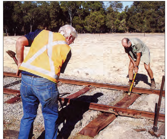
Duncan McVicar (left) and Trevor Dennhardt inserting a steel sleeper in the track north of Red Dam on 15 May. Lindsay Richardson
