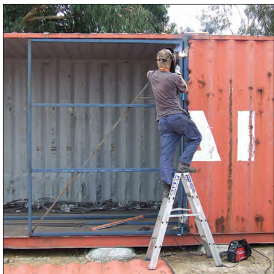
Frank Schroeders welds the frame for the doors on the motor storage container. Anthony Smith
