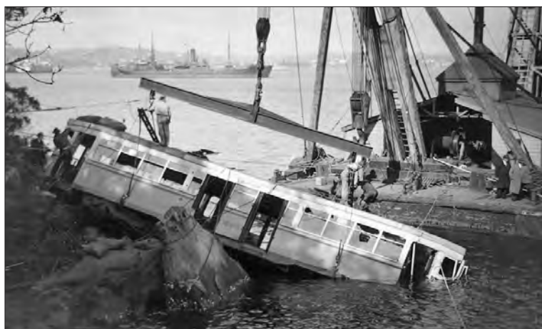
Bags of shavings have been placed on the roof at the rear of the tram and the rear trolley pole has been tied down out of the way. The bags of shavings were provided as packing onto which it was planned the car could roll while coming into a perpendicular position.
