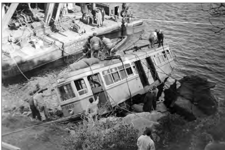
The tram is being prepared for lifting by floating crane
