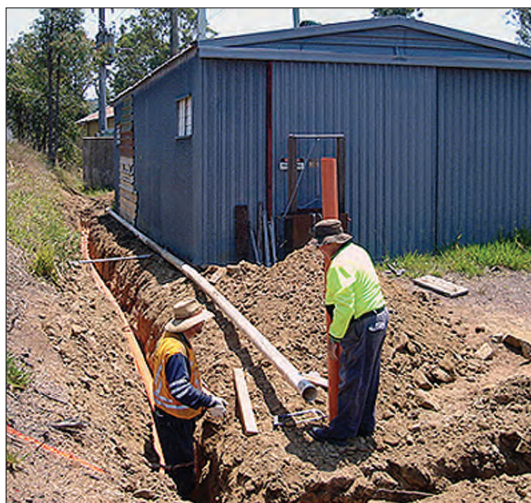
Ken Howard and John Lambert placing conduits for 11,000 volt cable. Peter Hyde
