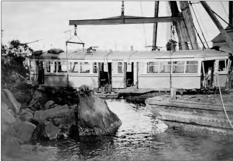
The tram is now level and the bags of shavings on the roof can be removed. John Burgess
