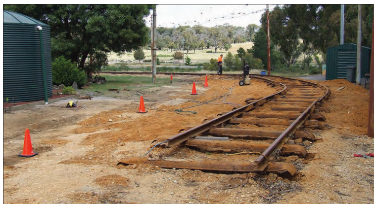
The south west curve is lifted to allow it to be levelled and realigned to match up with the north west curve. Jacqui Smith
