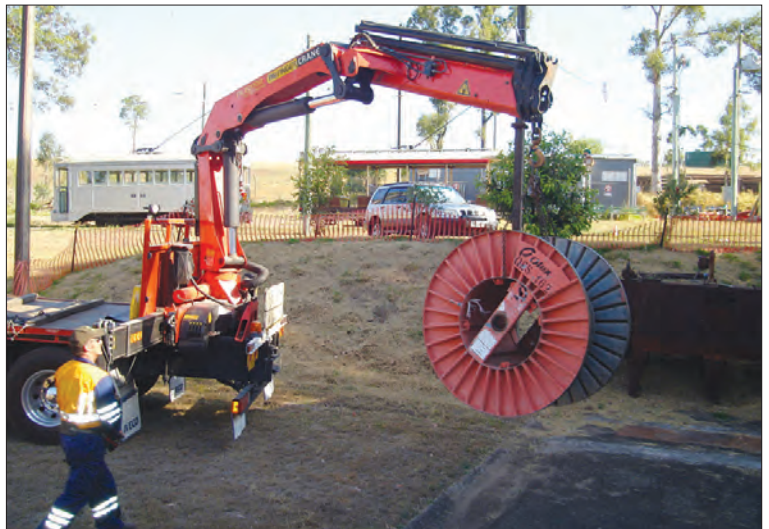
Delivery of 11,000 volt cable for the new traction power supply.
