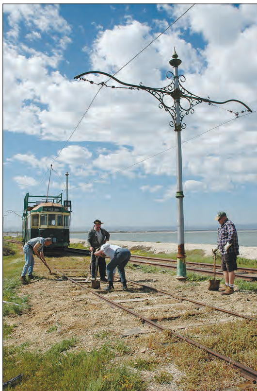
Greg Mayman, Ian Seymour, Jack Pennack and Steve Gordon repairing the loop track on 1 August. W2 354 is in the right of the picture.
