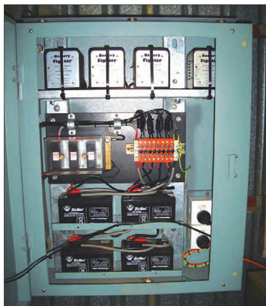
The new battery power supply for operating our 11,000 volt circuit breaker. Peter Hyde
