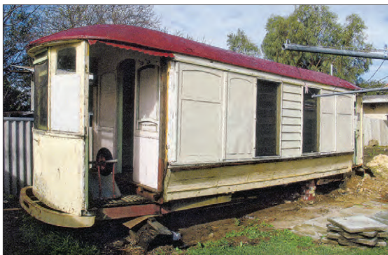
After the removal of the gabled roof, the side sheeting and the lean-to structures, the shed has been transformed into a tram in late July. The four glazed saloon windows are clearly visible, also the jarrah log support complete with white ant cap metal sheet at the near corner.
