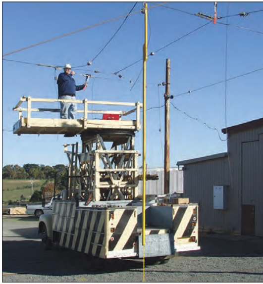
Kym Smith installs the new anchoring spans for roads 1 and 2 Anthony Smith
