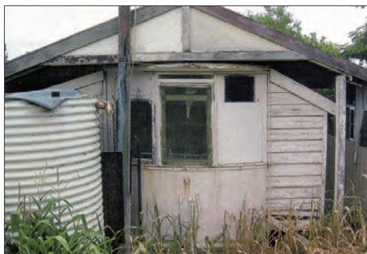
One end of B 43 as first seen in May 2009, showing the gabled roof that protected it so well. The weatherboard lean-to structure at right contains a cupboard opening into the end platform, where a sink was installed. Plumbing can be seen on the car apron.
