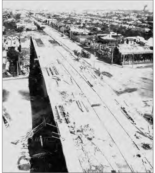
Concreting the deck of the Bakewell Bridge, 9 April 1925. An F type car can be seen entering Henley Beach Road from Deviation Road.
