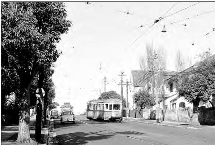
Two crossovers were provided at the terminus in Ocean Street which was on a moderate grade. A tram drifts through the upper crossover at the start of a trip to the city.
