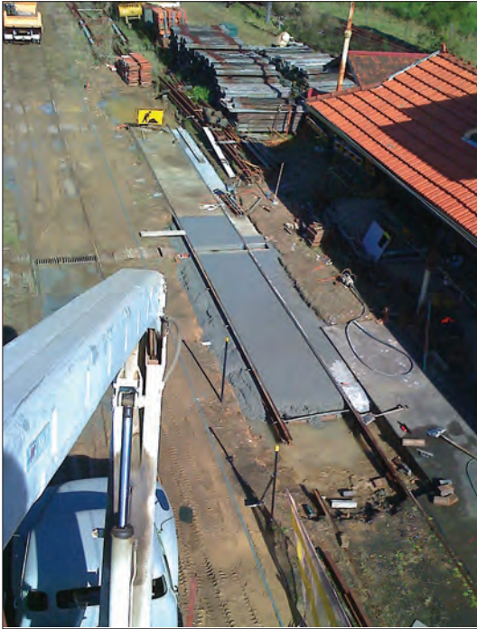
Five cubic metres of concrete was laid on 10 July on the western track in front of the Railway Square waiting shed including the track drain surrounds. This was laid approx 40mm lower than railhead north of the track drain to allow for bitumen topping.
