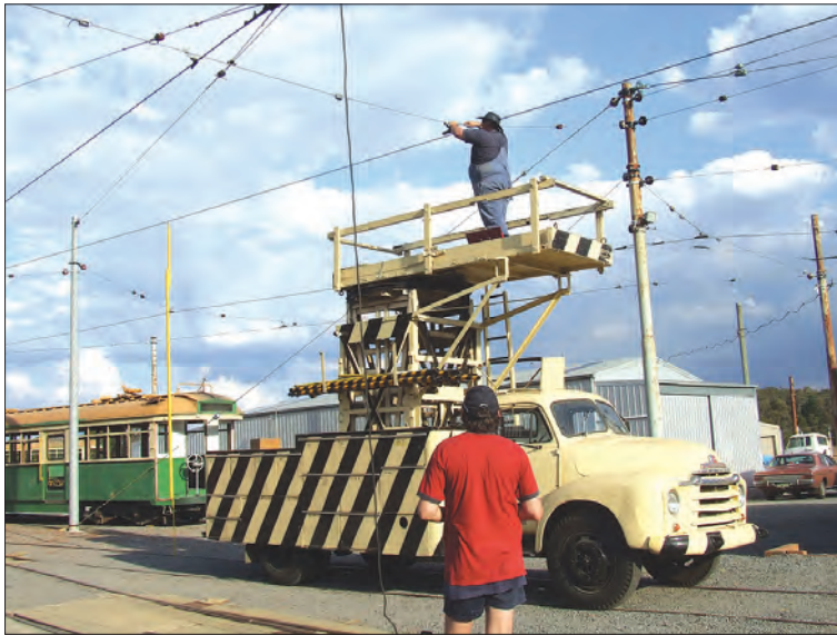
Anthony Smith watches as Kym Smith reattaches the ear to the new span from pole 7.
