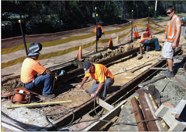
The installation of grooved rail in Tramway Avenue continues. This view was taken on 2 May.
