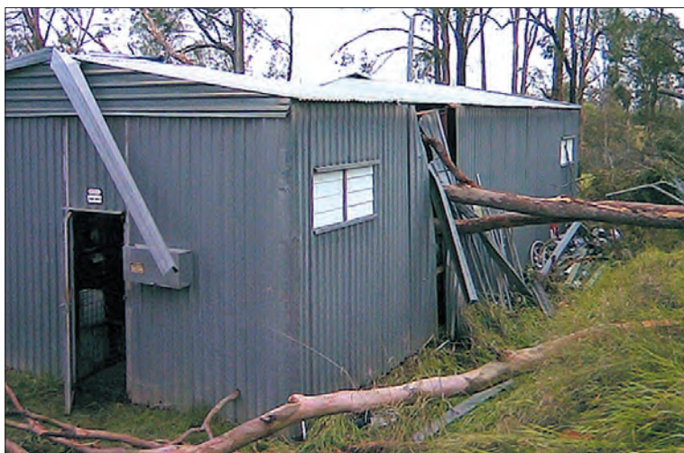
The tree that hit the substation. Glen Dyer
