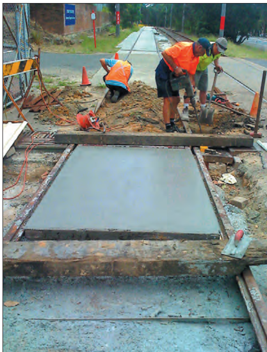
Rail replacement and concreting at the front gate on 8 November 2008.
