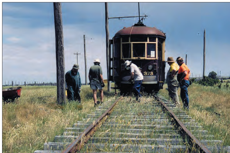
Assisted by H373 the track gang prepare to replace another sleeper on our main line.
