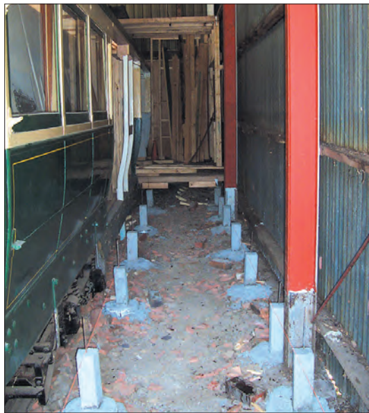
Work to reconstruct the display area along the north wall continues. New foundations were provided recently.
