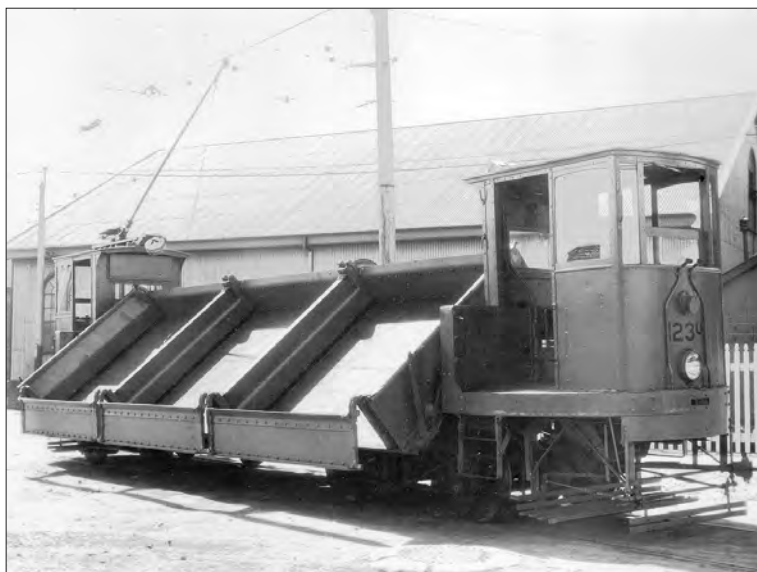
The car in the dumping position, with the bins facing the camera. R. Merchant collection
