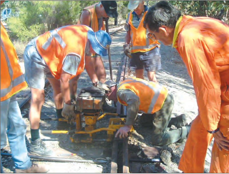
Installing the new checkrail on the Village Junction Curve on 29 March – Lindsay Richardson (left) and Noel Blackmore operate the modified rail drill to drill holes for the bolts securing the rails to the spacer blocks, as Trevor Dennhardt (behind Lindsay) holds the check in position; John Davies and Frank Edwards look on with great interest. Ric Francis
