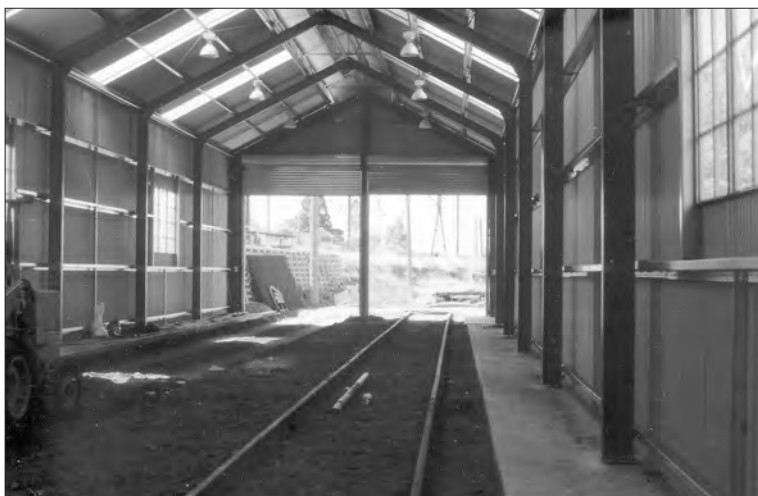
The original 80- and 90lb rail on timber sleepers has been replaced with 107lb on concrete sleepers. The second track has yet to be constructed.
