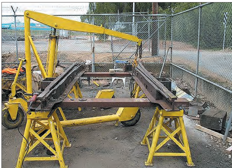
The Mundy Street points being fabricated in the yard behind the depot.
