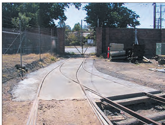
The Weeroona Depot points have been set in concrete.
