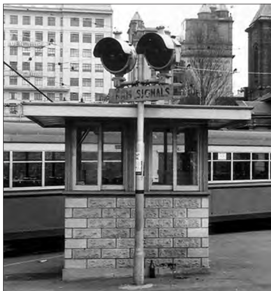
The Queen's Square signal box. The two tramway signals controlled access to St James Road and the tramway loop. Vic Solomons
