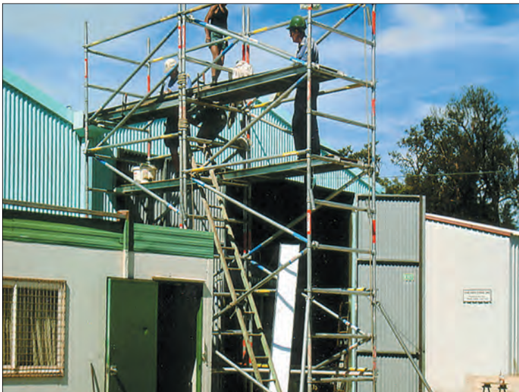
Work progresses on installing the new overlay guttering in the centre of the Oketon Geddes Car barn roof on 12 April. On the scaffolding at the western end of the building, Bryan Adcock, Trevor Dennhardt, Graham Bedells (obscured), and Frank Edwards prepare to process the next 3 metre length, which can be seen beside the ladder, below.
