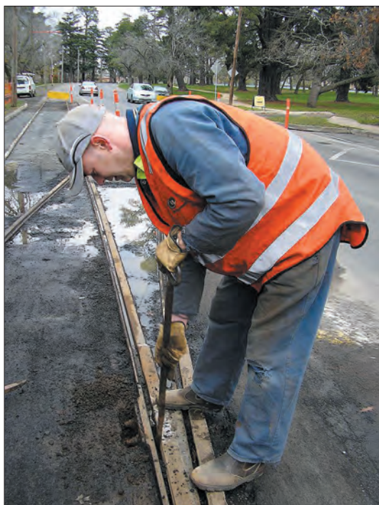
Garry Wood works on a point blade, 23 June 2007. Austin Brehaut
