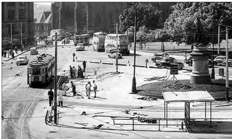
An R1 class car passes the new loop on 4 December 1950. Track laying has been completed and fencing and shelter construction is under way.
