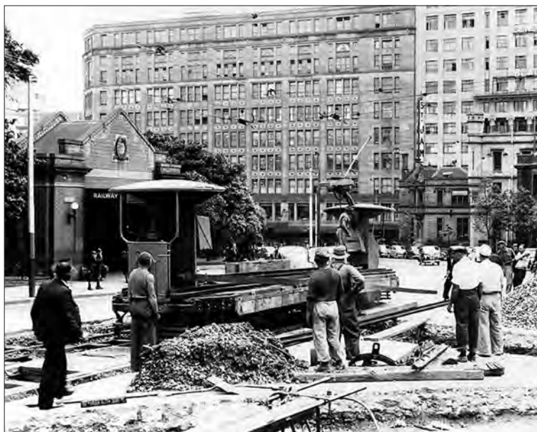
A ballast motor carrying rails during the construction of Queen's Square loop. The work started early in October and the loop was completed and tested on 7 December 1950.
