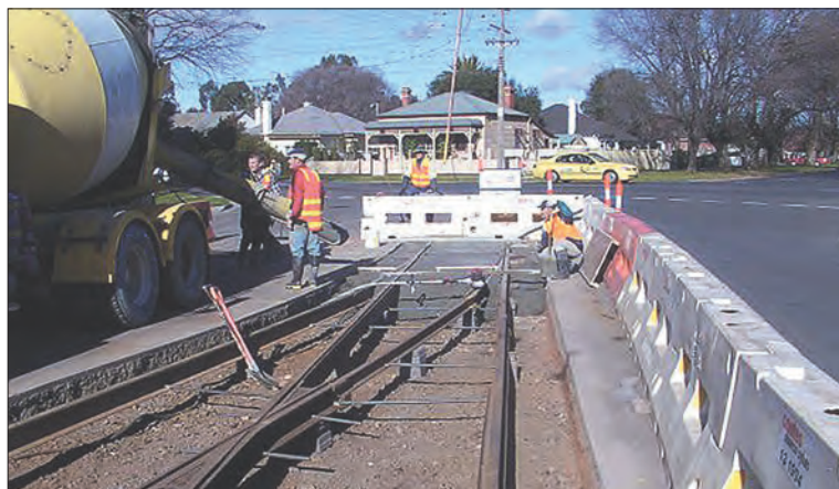
Concreting the southern set of points in Thunder Street. Bendigo Tramways
