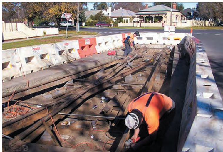
Karl and Sam work on the set of points at the southern end of the loop.
