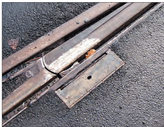
The new box made up to contain a point blade heel block, 30 June 2007. Warren Doubleday
