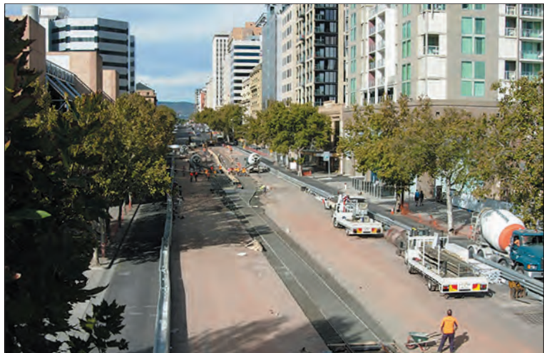
The same view taken on 8 April 2007 from the Morphett Road Bridge. The single track approaching the terminus (behind the photographer) allows for a traffic turning lane into the Adelaide Convention Centre.
