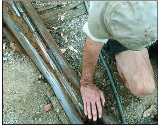
Noel Blackmore examines the failed crossing frog at the Stockmans Loop South points before its replacement on 7 February.
