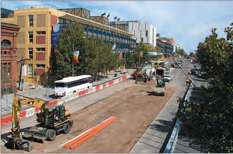
The road bed being prepared for the terminus at the University of South Australia's City West Campus on 7 April 2007.
