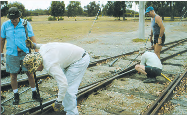
Trevor Dennhardt uses the rattle-gun to tighten fishbolts securing the new crossing frog in position at Stockmans Loop South points on 7 February.
