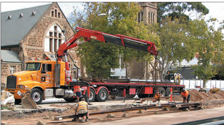
The first rails are laid, at 2:40pm on 7 April. At this point the double track converges to single as it approaches the terminus.
