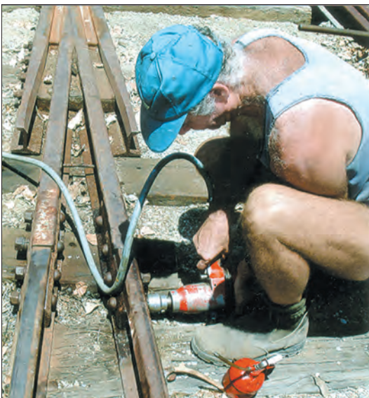
Trevor Dennhardt uses the rattle-gun to tighten fishbolts securing the new crossing frog in position at Stockmans Loop South points on 7 February.
