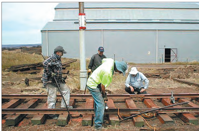
Graham Jordan (in yellow shirt) positions another sleeper prior to drilling and spiking. Paul Constantinidis, Andrew Hall and Geoff Dean wait for the next move, on 18 November 2006.
