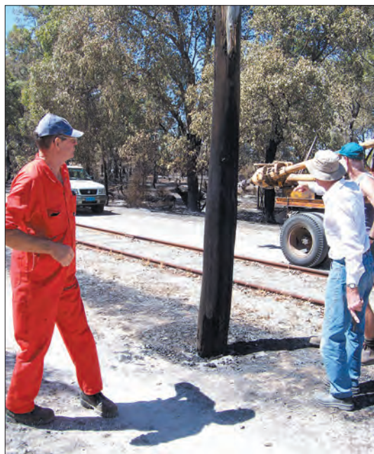
John Azzaro (left), Noel Blackmore and Trevor Dennhardt inspect the fire-damaged traction pole on 6 December. It was badly burnt at the base after an earlier attack by termites.
