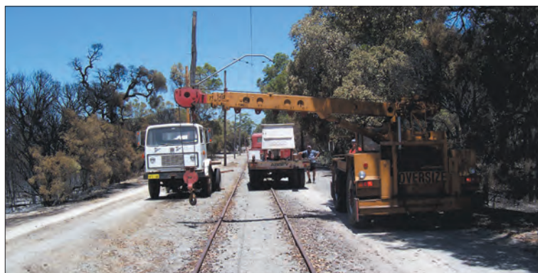
Frank Edwards operates the post-hole auger in preparation for the installation of the new steel pole.
