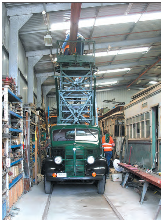
Overhead troughing being erected in the top shed with the aid of a tower wagon, 2 December 2006.
