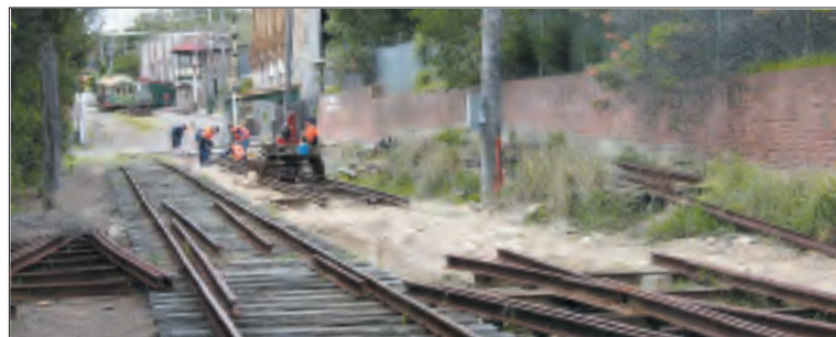
The trackwork continues in the cut leading from the museum grounds as seen on 21 October. The pointwork is on site and the second track is being reconstructed and will be concreted. Bob Merchant
