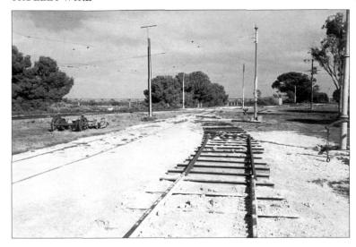
Work has commenced on the laying of Road 9 (right) into the Northern Depot. It branches off Road 10. The main line is further to the left. Ian Seymour
