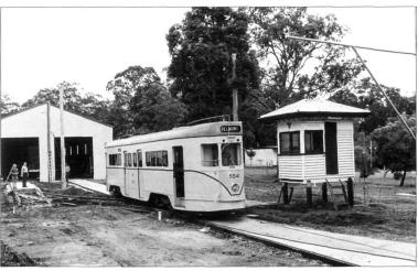
Noel West drives 554 past the signal cabin en route to the main running line. The bare area in the lower left is for the future shunt stub off the pit road (left) track in the workshops. The wandering lead is attached to the section of overhead between the two poles in front of the new shed.
