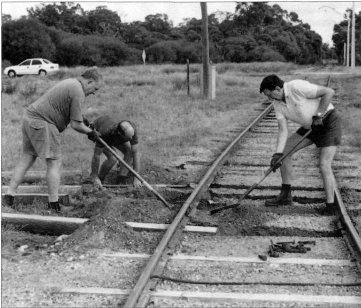
At Farmgate Curve on 16 May 1999, John Shaw (left), Trevor Dennhardt and Lindsay Richardson are installing the first group of treated pine sleepers for trial.
