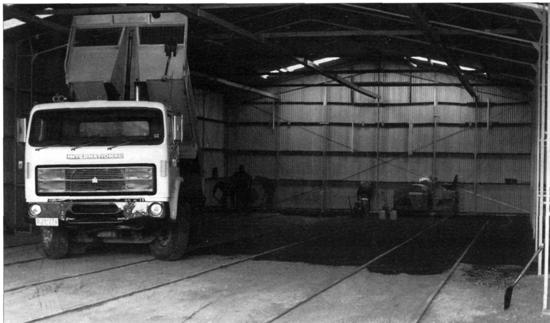
Bituminising the car barn floor in progress.
