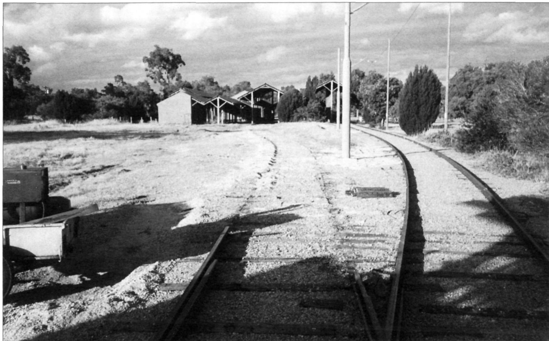
The bare trackbed of the inside road at the entrance at the end of the day on 22 November 1997. New steel poles support the overhead on the outside road (right).
