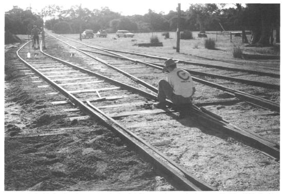
Andy McCutcheon's team apply the finishing touches to the loop on 17 July 1993 (looking north). The left-hand turnout from the main line at the centre of the loop forms the present northern apex of Stockmans Crossing; it will be relocated south of the loop when the track at Stockmans Crossing is realigned.
