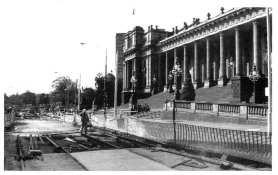
A view of Spring Street outside Parliament House on 18 September 1993. This missing section of track was laid and concreted over the weekend 18/19 September.
