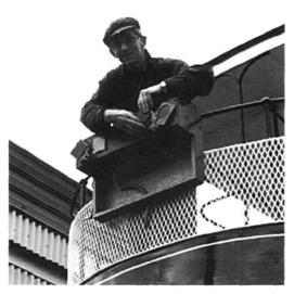
Kay Morgan replaces the coloured glass in the destination box. The coloured indicators were visible at night for a distance before the actual destination could be read.
