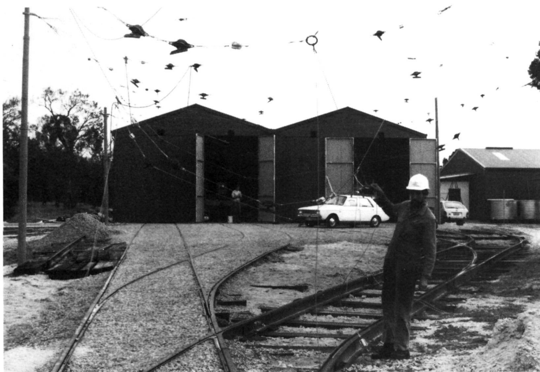
Frank Edwards assists with the erection of the web of wiring over the depot yard pointwork.
