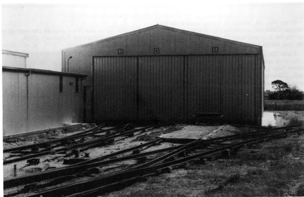
The depot yard track is shown assembled and levelled awaiting the pouring of concrete to form a mass roadbed. K. McCARTHY
