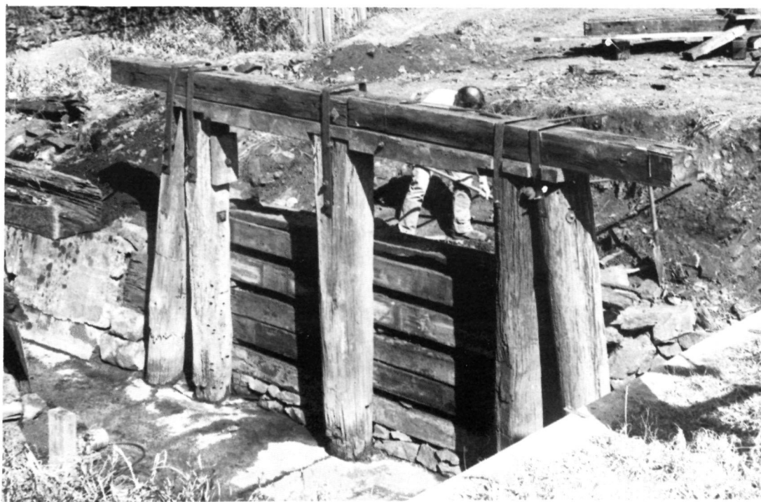
The reconstructed western abutment pier on the Mt. Keira Colliery tramway bridge over Smith's Creek in Osborne Park Wollongong on 9 August 1980. Prior to reconstruction the centre pier and the twin piers at the left were the only items remaining of the western abutment. -K.McCarthy
