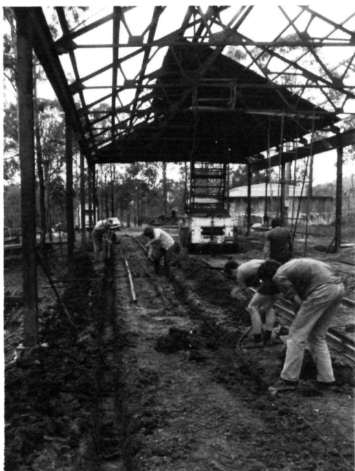
Laying the track while no. 1 depot rises above.
