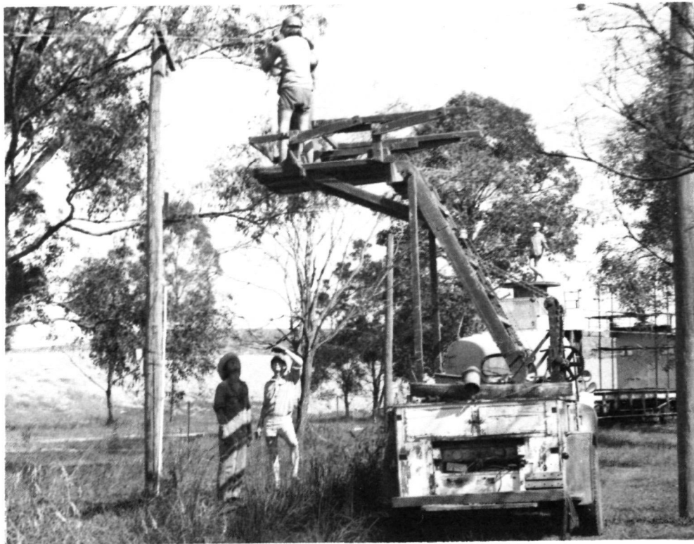
Erection of the overhead took two days, using tower waggon 1.
