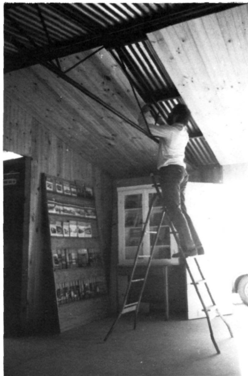
John Hoffmann is completing part of the ceiling lining in the visitors' entrance building at St. Kilda. - John Radcliffe
