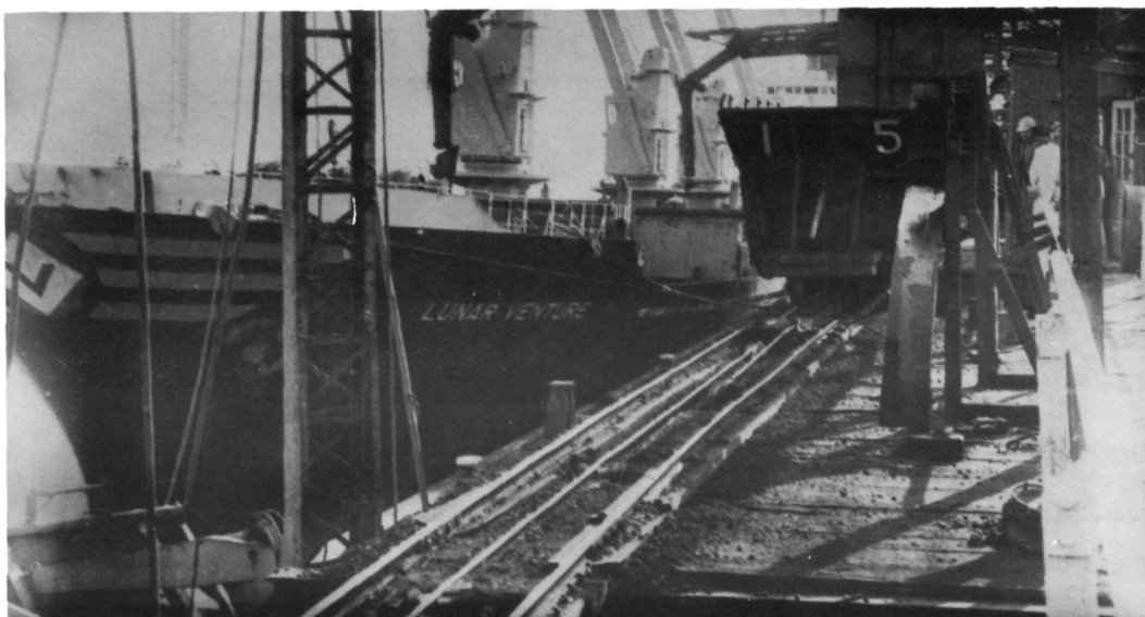
Loaded hopper wagon 15 passes over the weighbridge beyond the change of cable point, as the ship Lunar Venture rapidly fills with export coal. The cable railway only had another 24 hours of activity when this photo was taken on 3rd April.
