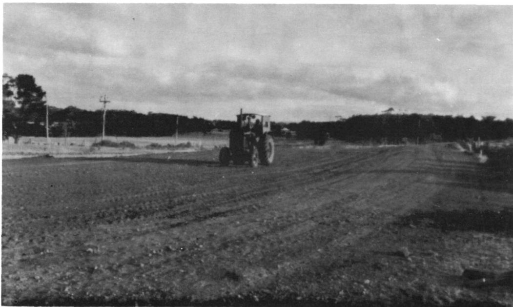
The hills of Bylands form a backdrop to the tractor being used to consolidate the earth of the carpark after levelling by the grader.
