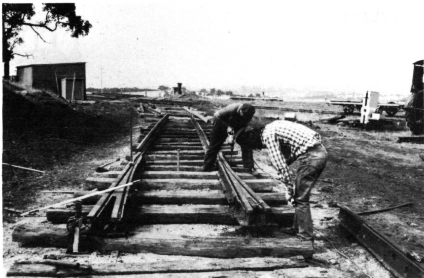
The first turnout under construction at Bylands, leading into Nos. 1 and 2 roads. This depot branch leaves the mainline beside the shed at left. 9th February 1975. —Keith Kings
