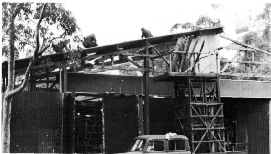
Bob Cowing, Mike Giddey and Dick Jones screw down roofing while Bill Denham, partly hidden by the floorboards stacked on the tower wagon, nails the vertical boarding to the gable.
