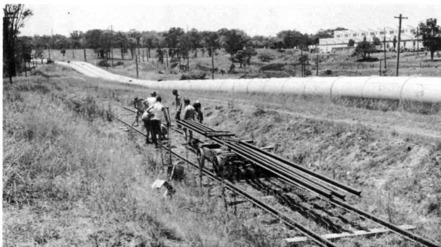
The end of a railway line: rails from the Potts Hill track removal project are loaded onto the trolley on 22nd January.
