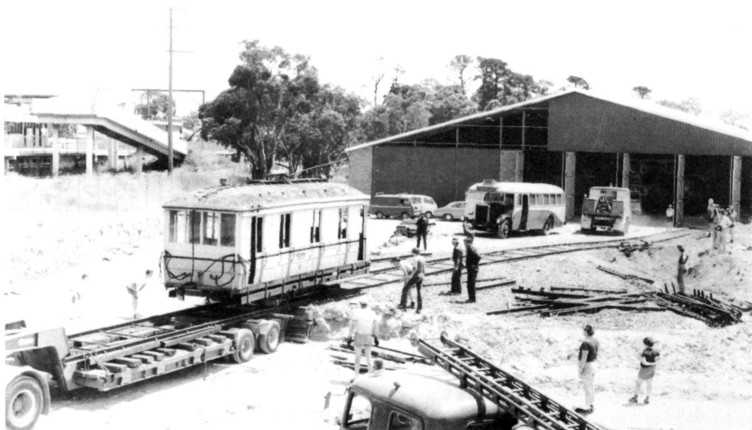
E529 being winched off the lowloader by the Matador tramcar recovery vehicle at the Loftus site on 20 November, 1982. Loftus railway station can be seen to the left of the depot building.
