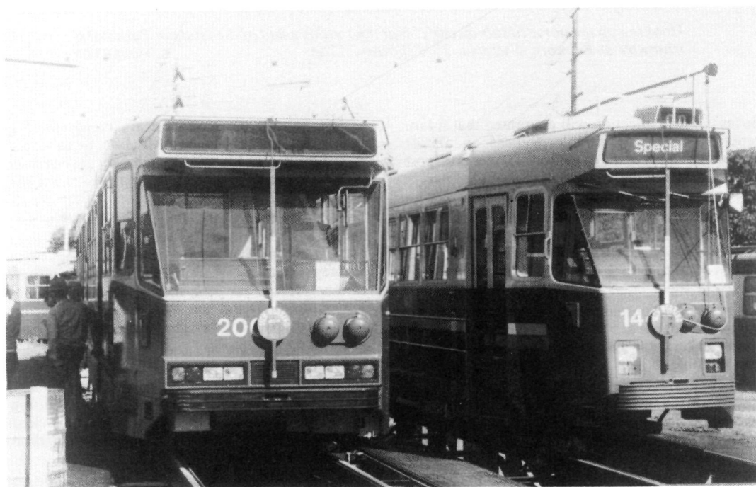
A comparison of front ends. Articulated car 2001 (left) and Z3 car 144 at Preston Workshops. "Men Working" signs hang from the destination box rails on both cars.
