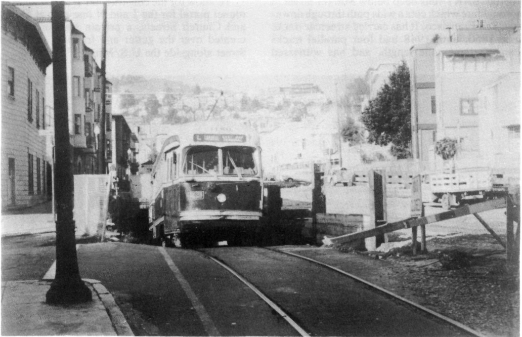
Ex Toronto PCC 1180 rises to the surface of Market Street from the temporary portal of Twin Peaks Tunnel. The new Metro tunnel joins into the Twin Peaks Tunnel at this point and the nearly completed construction work is to the right of the tram.
